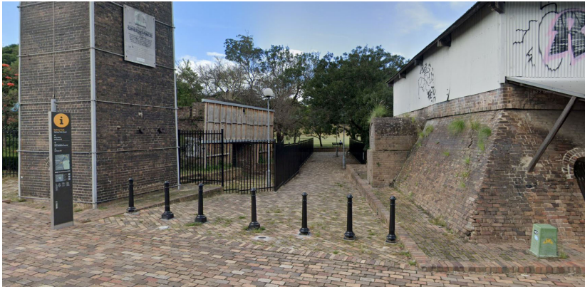
Main pedestrian entrance to kilns
